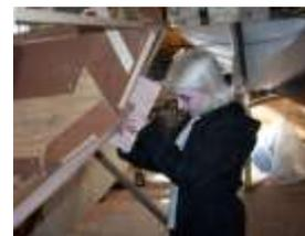
student for a couple of days. Chloe had come over to see us from Belfast. Over left at the bottom of the previous column she is marking the hull of the skiff with a gauge to show the plank land..
