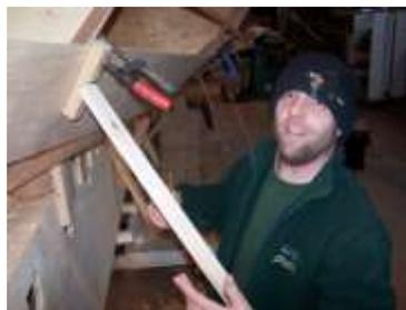
conjunction with a set of dividers to mark off a series of points along the full length of the boat to take off the shape the shape of the new plank. Once marked the spiling plank is laid onto the full plank stock and the lines are taken off. Below left Alan Beattie (2) and Dave S are giving the position a final once over. Below right is a photo of Marian taking a photo along with Jim who is doing an impression of the ‘Man from Delmonte’
