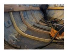
we could pull in the forward plank. In the photo over right John P and Trevor D are cutting a rebate to take a full length biscuit to glue up two halves
