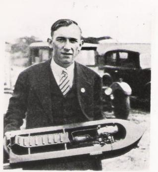
Mr. A. W. Martin, of the Southampton Model Power Boat Club, with his flash steam hydroplane "Tornado II," fitted with coil boiler single blowlamp, and single-cylinder piston valve uniflow engine. Weight 4 lbs., speed 24 m.p.h.
